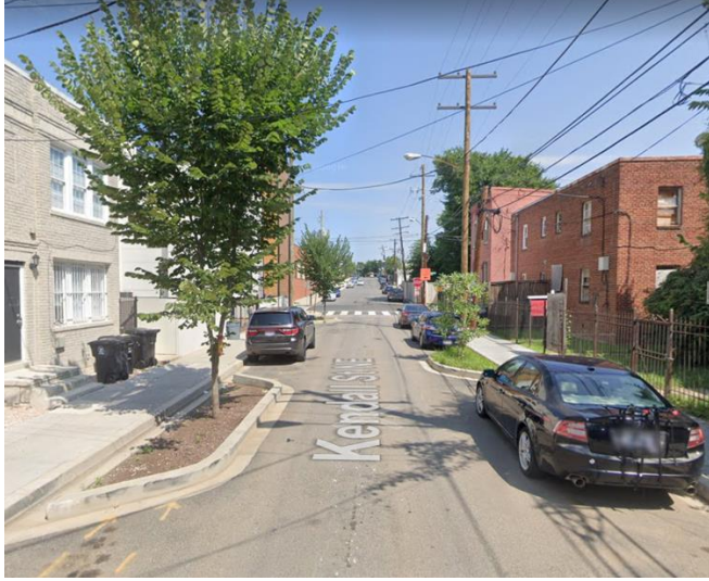
Recent DDOT project in Ivy City
